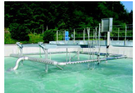
Fig. 1: Final clarifier of a sewage clarification plant 1)
